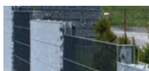
Column with integrated U-rail.
